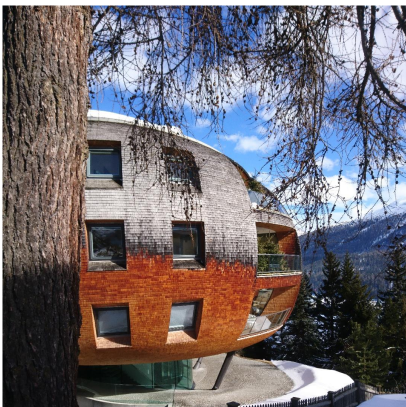
Fig. 2: Chesa Futura, St. Moritz: Norman Foster demonstrates the elegance of a Minergie-P insulation (≈ 30 cm) – and with 50 cm even more than Minergie-P. “ The elegance of an insulation does not depend on the bulky of the insulation, but on the knowhow of the architect. ”
