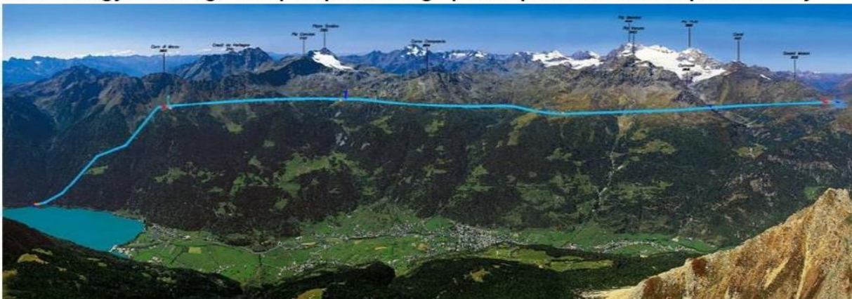
Fig. 9: The 1.05 GW PPT planned on the Bernina/GR costs around CHF 2.5 billion; the same battery storage capacity for a comparable service life of 80 years would currently cost around CHF 25 billion. (cf. PEB building study 2019; Part I lit. C no. 1).
